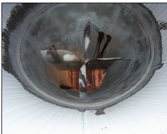
Figure 9: Photograph of digester cone and cross-piece baffle.
