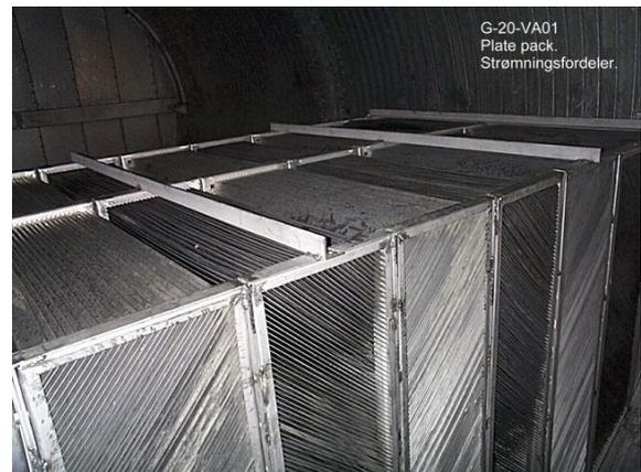
Figure 3: Photograph of parallel plate arrangement.
